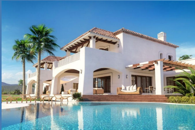
Villa Automation Solution
