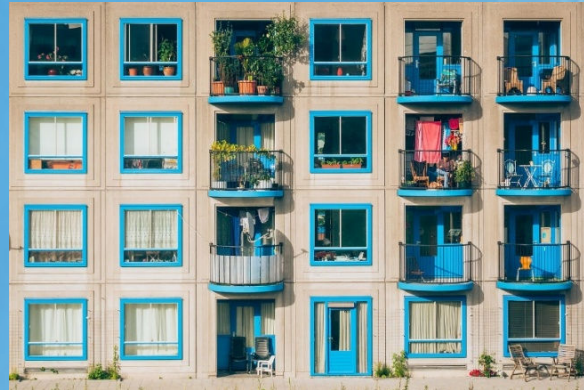
Apartment Automation Solution
